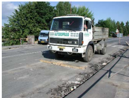
Fig. 4 Bridge structure loading
