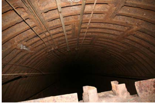
Fig. 2. Inside view of investigated shaft
