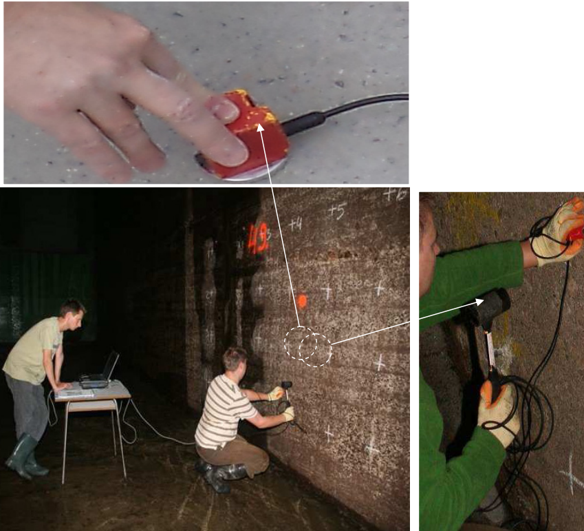
Fig. 1. Testing of massive structural element, i.e. concrete wall of hydroelectric power plant suction pipe, by means of impulse response apparatus.
