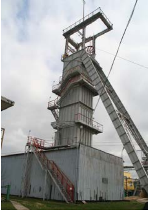
Fig. 1. Outside view of investigated shaft.
