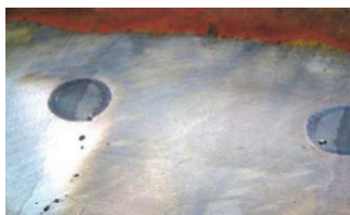
Obr. 11 Detail svaru, ventilu
